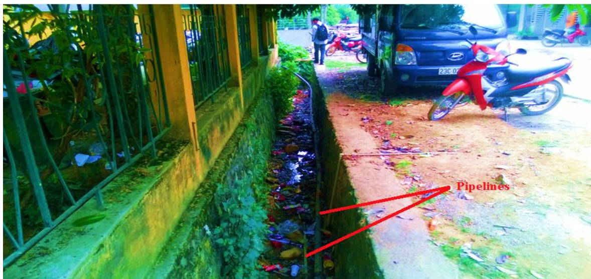
Figure 5.31. The picture of pipeline inside wastewater near test point 5 (zone 9)
