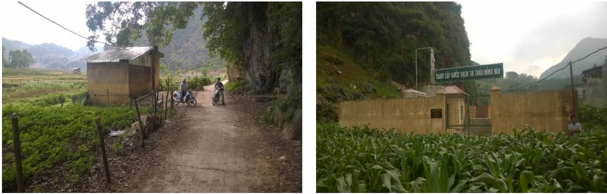
Figure 5.2. Lang Nghien and To 5 pump station
