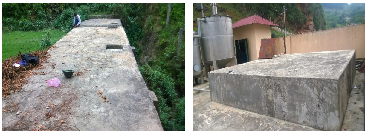
Figure 5.6. Tank 5 at Xom Moi (left) and tank 2 at To 5 pump station
