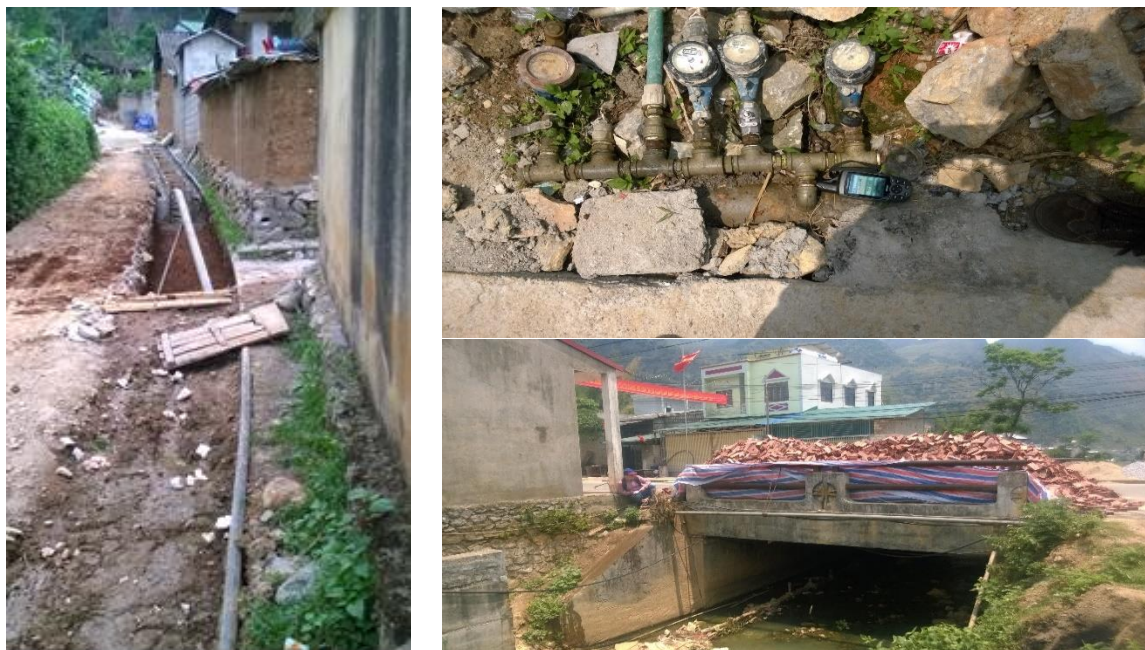
Figure 5.4. Pipelines in central city
