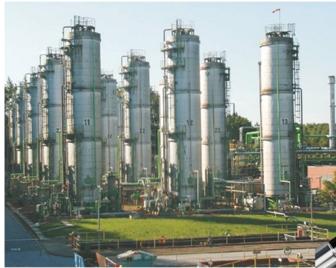
Production of 600,000 t/a phenol in 15 bubble columns by INEOS Phenol, Gladbeck, Germany
