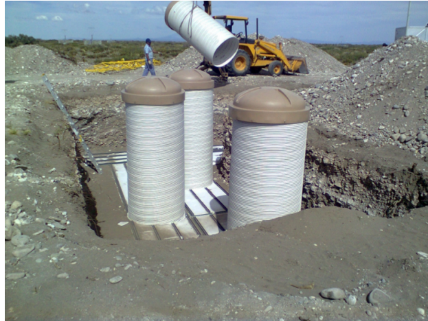
Figure 1.8: Installation of one of the 30 m 2 buried, scintillation-based muon counters. These counters will directly measure the muonic component of EASs approximately at and below the energy of the spectrum’s ankle. Picture from [15].
