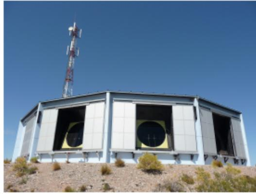
**Figure 3.3:** Two different view for a FD building. Schematic layout (a) with six fluorescence telescopes from [66] and a daytime photo of Los Leones FD telescopes (b) the shutters were opened for maintenance from [63].
