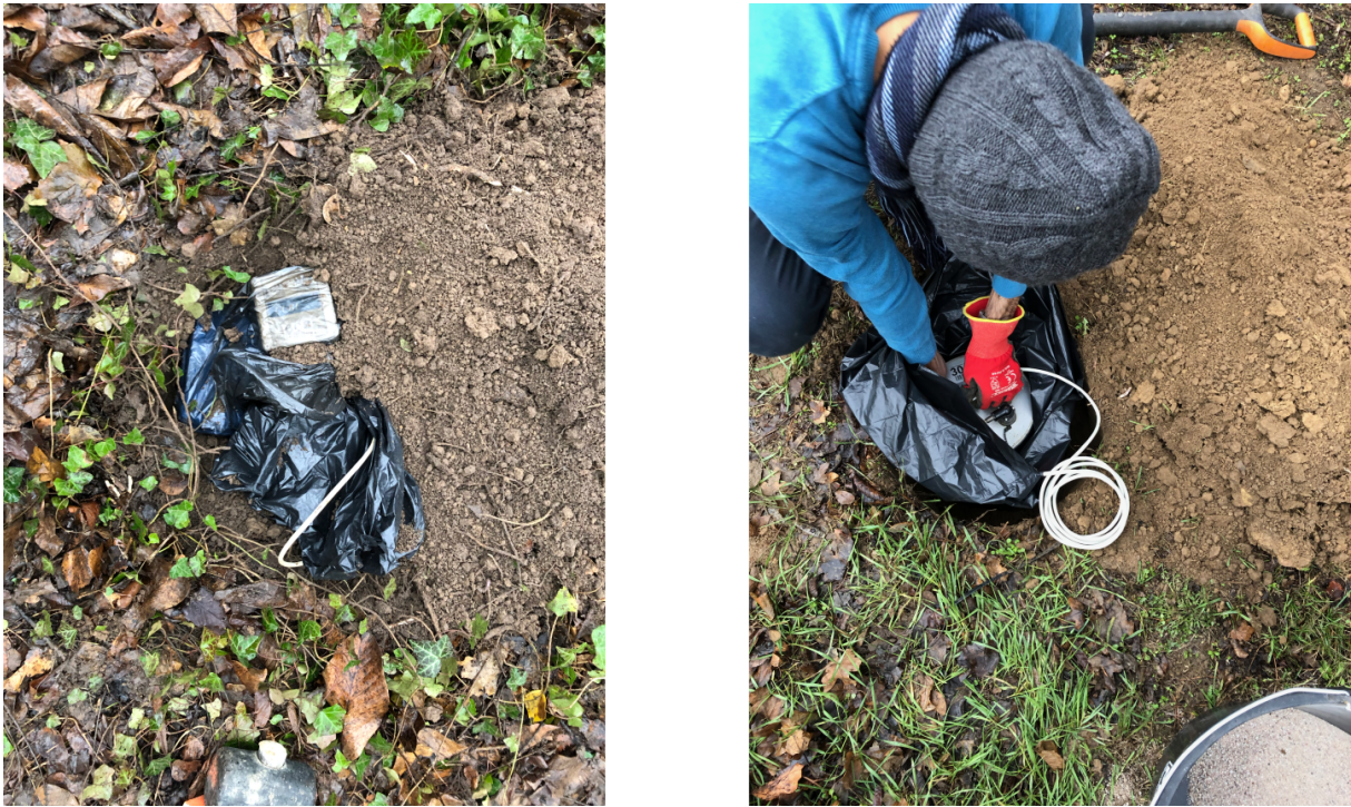
Figure C.2: Exemplary instrument installations at recording station S1D3. The sensors were protected with plastic bags (black) against moisture and buried to a depth of about 30 cm. Left: Buried sensor inside the plastic bag. The CUBE3 data logger is located at the surface to ensure a stable GPS connection. Right: The seismic sensor during the installation.
