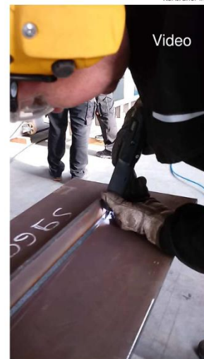
HIFIT treatment of a fillet weld
