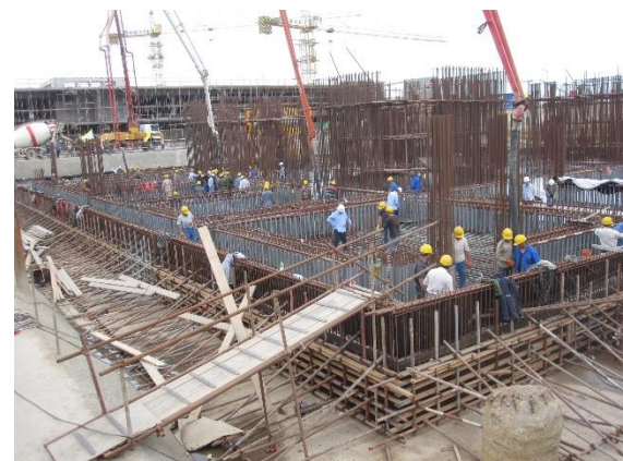
Abb. 16: Betonage Bodenplatte d=3,0 m Minarett [16]
