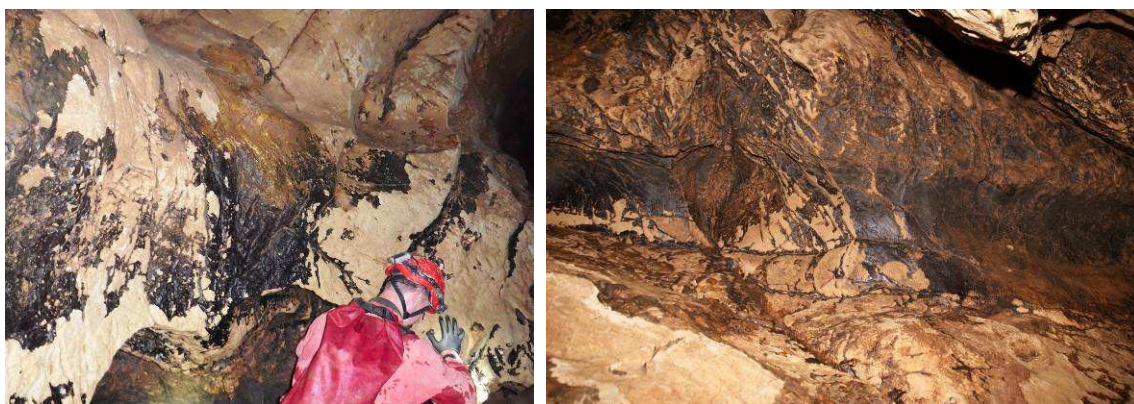
Figure 3.30: Black crust on the walls of cave Sang Ma Sao (left picture taken by Lai Quan Tuan (VIGMR) on March 12 th , 2014; right: March 27 th , 2016).
