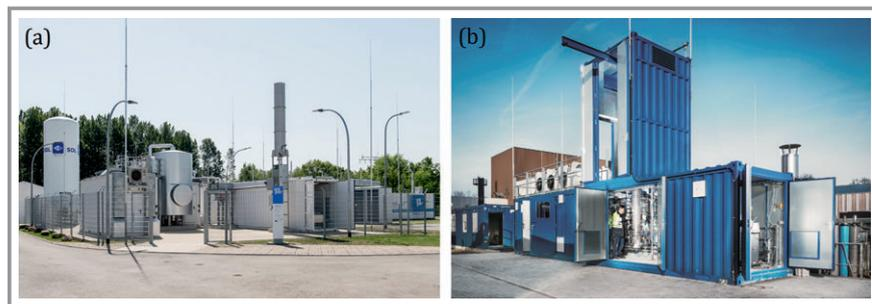
**Figure 6.** HCR plant with 1 MW installed electric power in Falkenhagen (a) and SBCR plant with 100 kW CH<sub>4</sub> output in the Energy Lab 2.0 (b).
