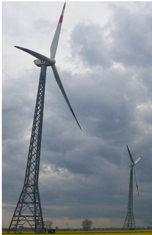
Figure 2.12: 2.5 MW rated power WTs with 100 m rotor diameter and 100 m hub height mounted on a Butzkies lattice tower in Bahrenfleth, Germany. Photo: A. Struve 2018
