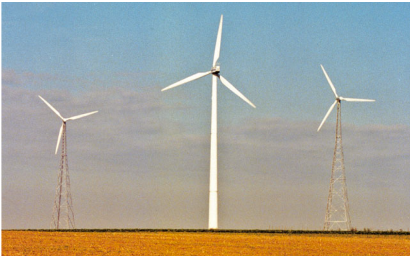
Figure 2.25: Subjective visibility comparison between conventional tubular steel tower and lattice towers. Photo: Sinning and taken from Hau [93, p. 520]
