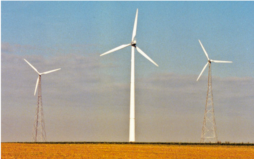
Figure 2.25: Subjective visibility comparison between conventional tubular steel tower and lattice towers. Photo: Sinning and taken from Hau [92, p. 520]
