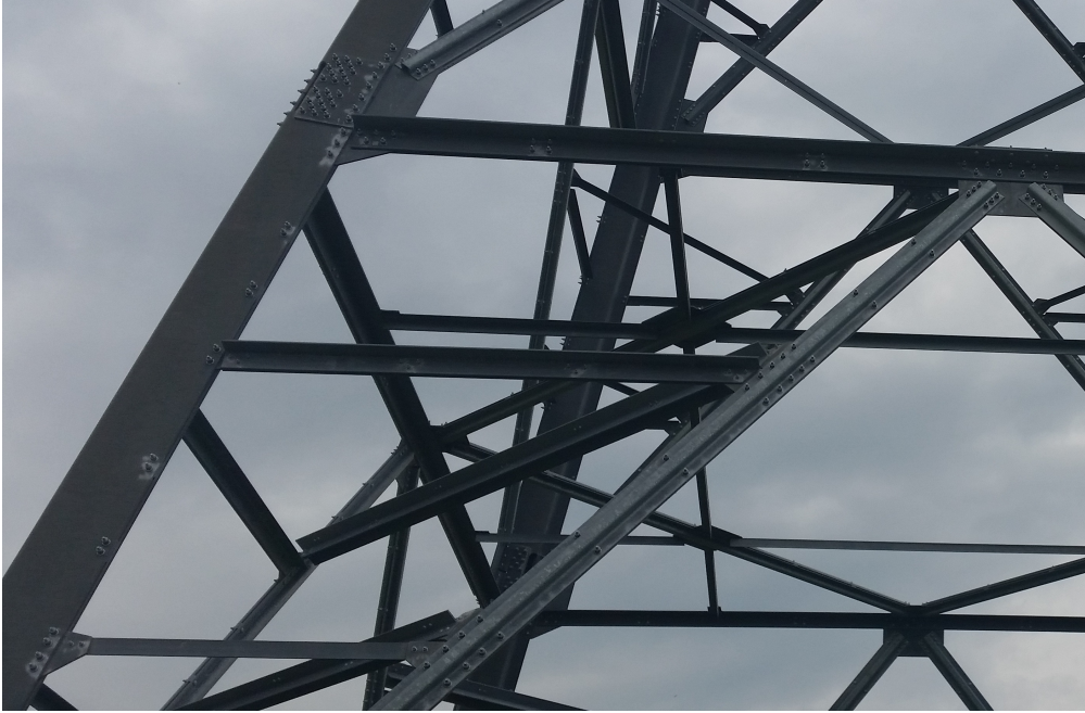
Figure 2.19: Different joints of a Butzkies lattice tower. Photo: A. Struve 2018
