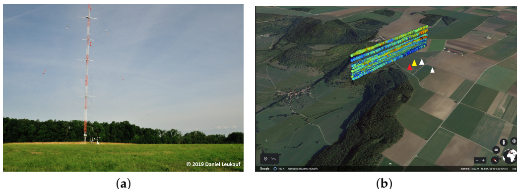
Figure 2. (a) View of the tower taken from east-southeast. To the west the tower is a dense canopy. This picture shows that the lowest anemometer (10 m) and the EC-station are directly downslope of the forest; (b) the flight patterns performed over the two days in September 2018. The colors along the legs indicate the measured horizontal wind speed. The red triangle marks the position of the tower and the yellow one is the EC-station. The white triangles are the future locations of the wind turbines.
