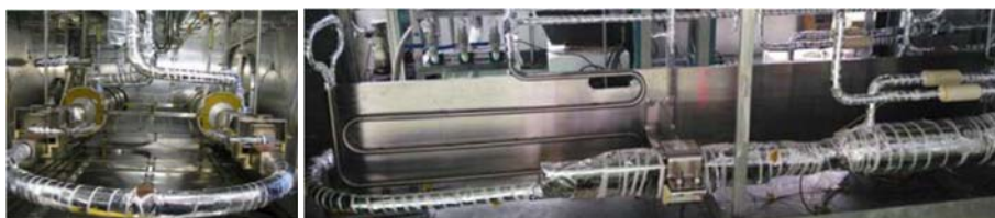
Figure 4. TF current leads installation in the test cryostat.
