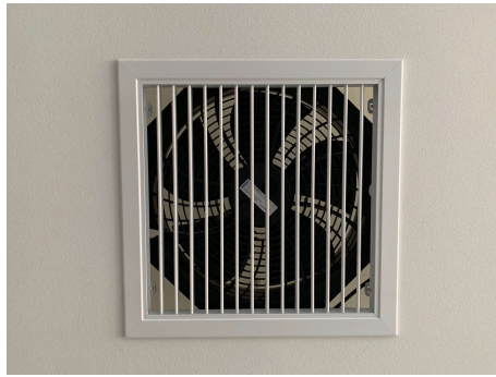
(a) View from below: mounted grille with an angle of 90°
