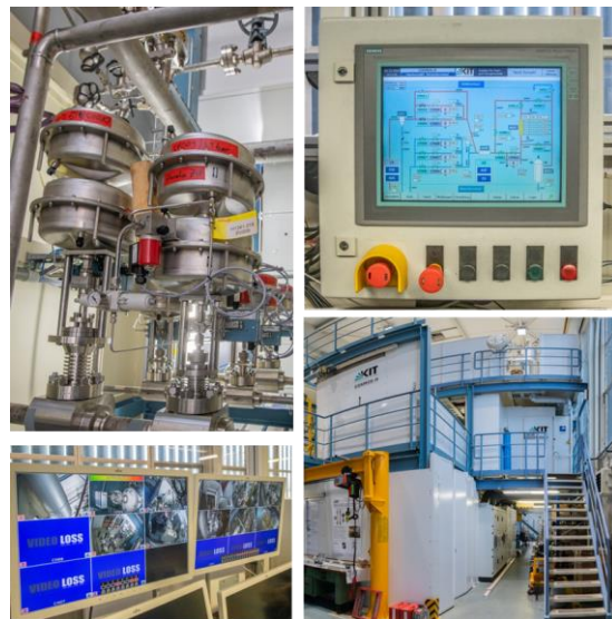
Figure 6: Images of various subsystems of the plant under construction
