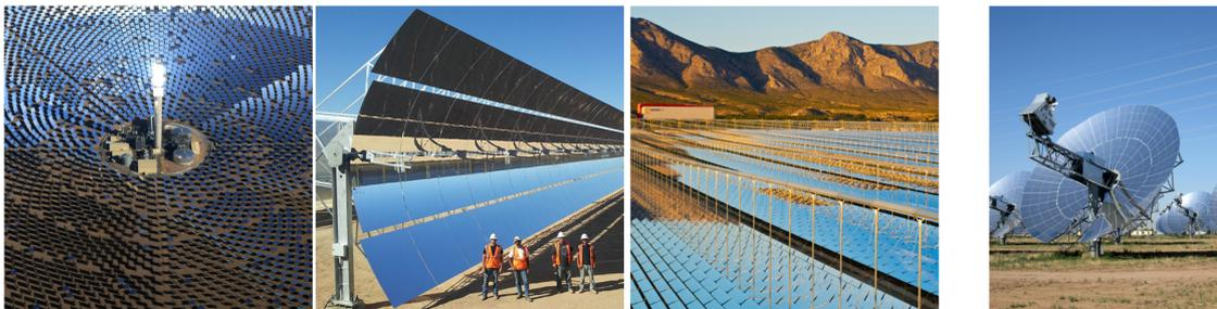
**Figure 2.3:** Some examples of solar field and solar collector configurations (from left to right): solar tower (courtesy: Solar Reserve), parabolic trough [101], linear Fresnel (courtesy: Novatec Solar) and solar dish (courtesy: Tessera solar).
