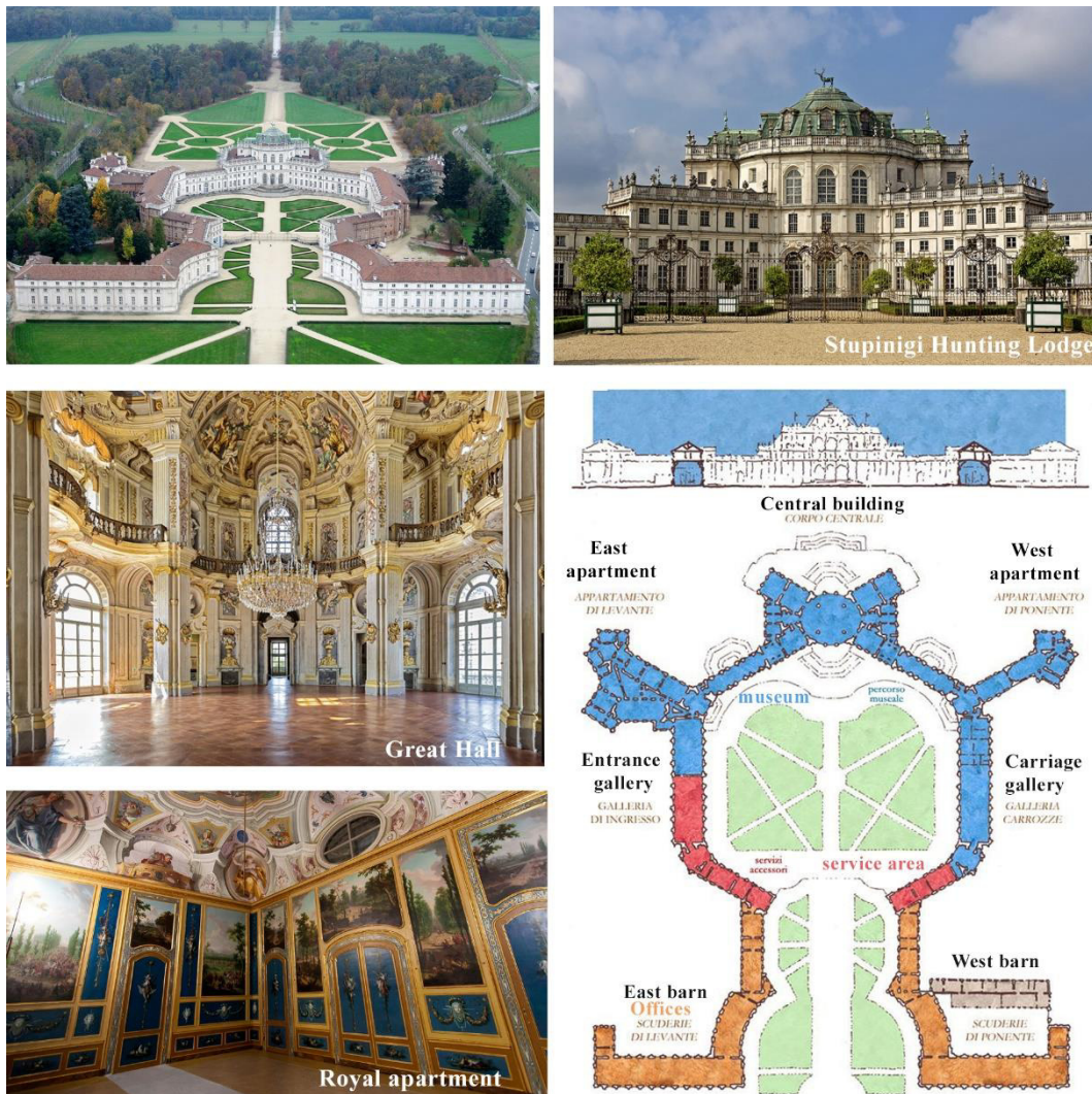
Figure 120. Stupinigi. Photos of the hunting lodge and the restoration project.
