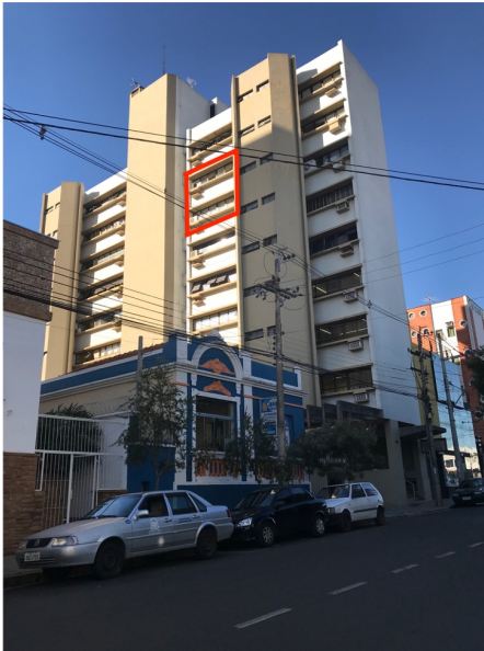
(a) Building where pre-test took place
