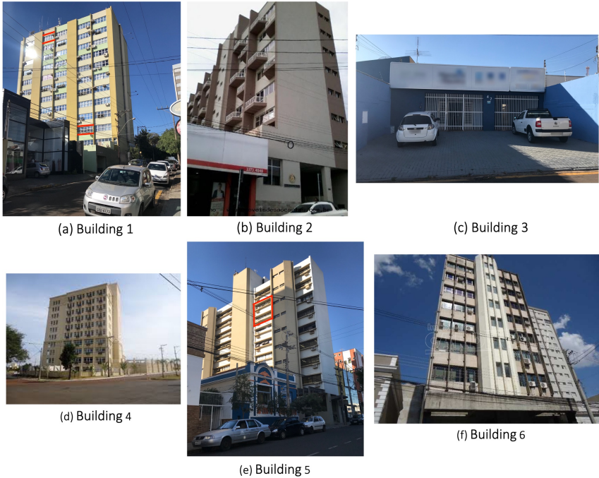
Figure 3.4: Buildings in final data set.
