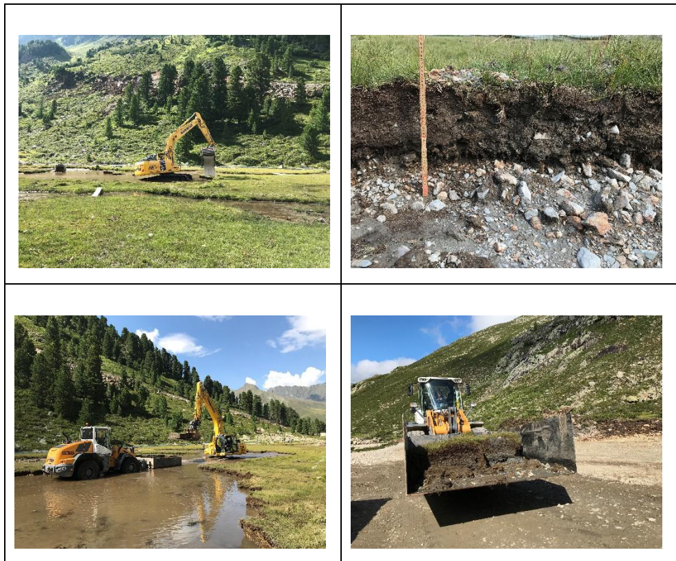
Fig. 2. Transplantation of an alpine Carex fen: Workflow at the donor site. (a) extraction of the turf at the donor site, (b) mean thickness of the turf was about 40 cm (based on fluvial gravel), (c + d) each piece was transferred immediately onto a wheel loader
