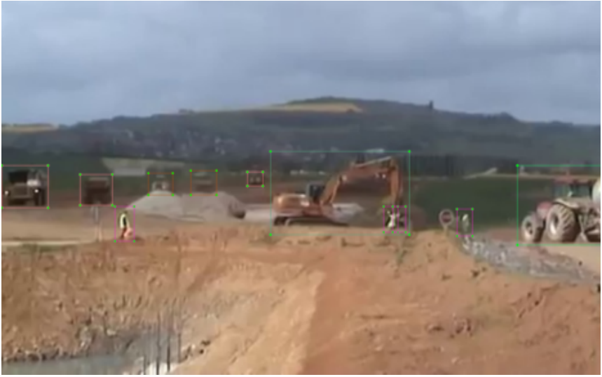
Figure 6.7: Label example. Rectangular correctly encompass ground truths: a dumper, an excavator as well as two persons. However, other trucks can be inferred from context stream frames but are not identifiable in the single image. The label should be ignored if YOLOv3 is used to detect mobile machines.
