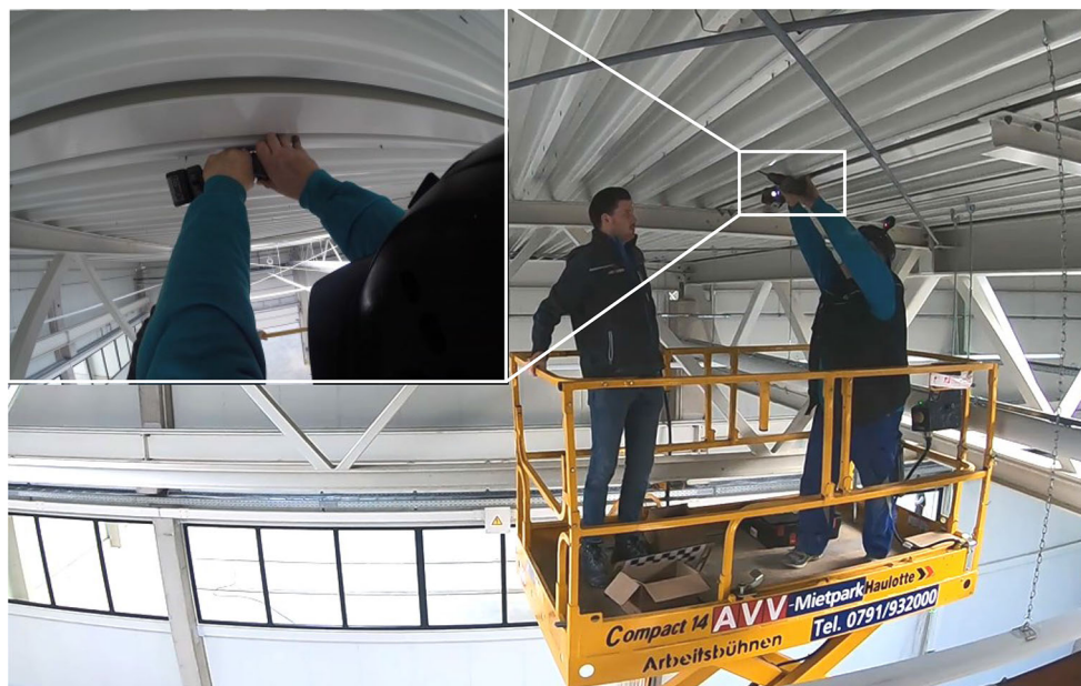
Fig. 6 Installation of cable clamps recorded in the long shot and from the users view (left corner)
