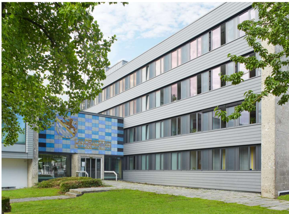
Figure 3: Main district building east façade (DBW-Architekten)
