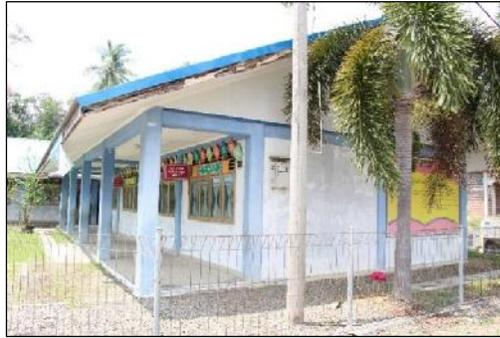
Figure 4.4: Verandah (corridor) and long roof span to minimize solar heat gain
