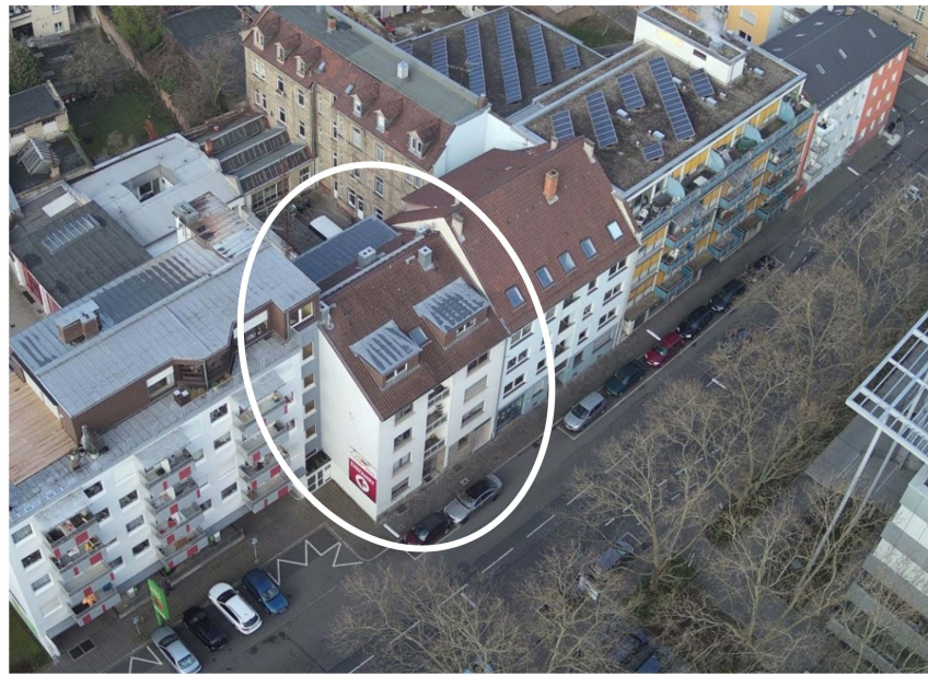
Figure A29. Reference building for an exemplary thermal bridge assessment (north orientation).
