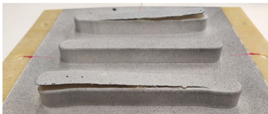
Figure 4.53: Damage pattern of the CoDiCo demonstrator part reinforced with UD-tapes in the top chord. A speckle pattern was applied for optical measurement of the strain field with a Digital Image Correlation System (DIC). 40
