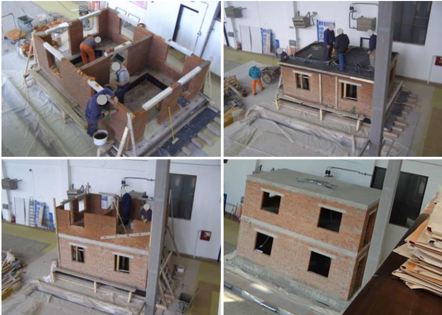
Figure 6.2: Construction of the BM model [73]
