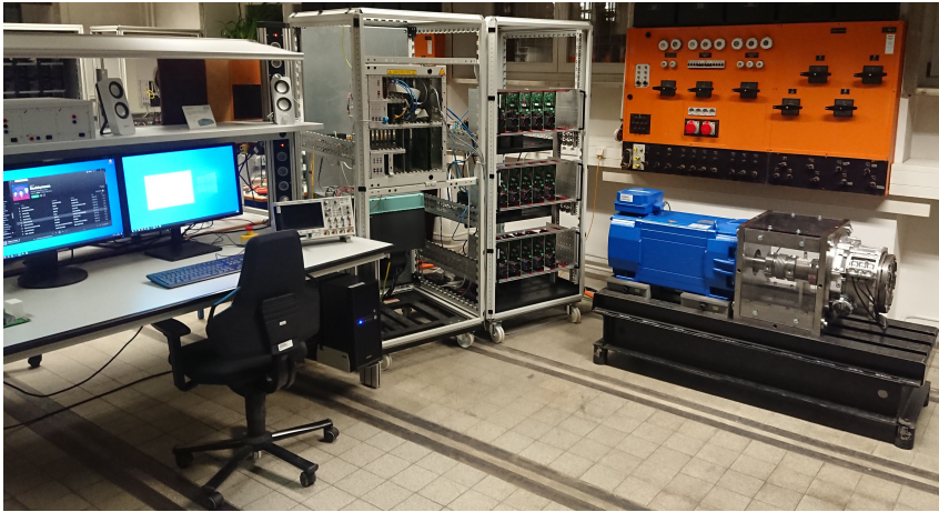
Figure 6.17: The prototype MMSPC, including the motor test-bench, control cabinet and HMI
