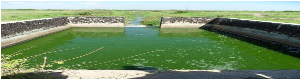
Figure 3.17: Green effluent due to high amount of algae in Ruai treatment ponds, Nairobi, Kenya
