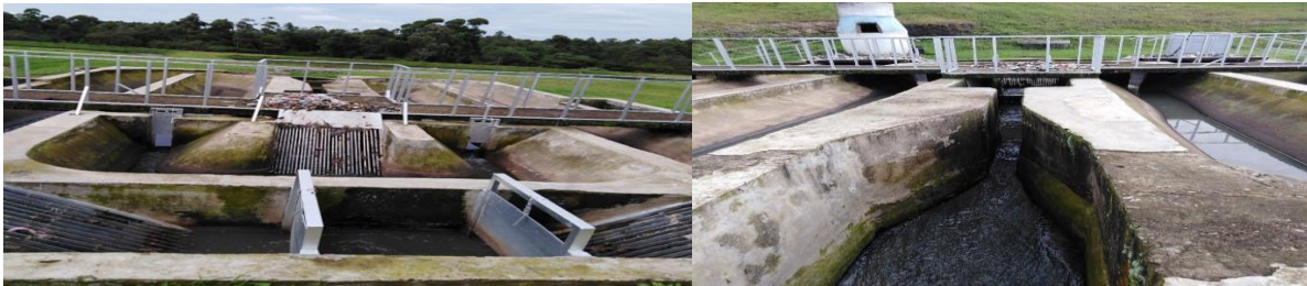
Figure 4.23: Intake point at Bomet wastewater ponds system
