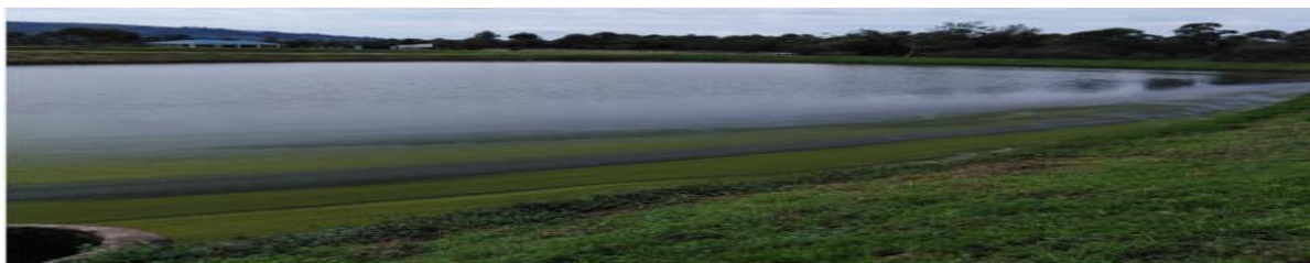
Figure 3.5: Thin surface layer of algae at Bomet wastewater ponds system, Kenya
