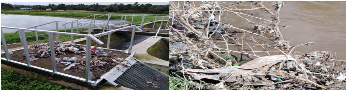
Figure 4.8: Building up of non-biodegradable (solid) waste at Bomet WPS (left) and Nyangores river (right)
