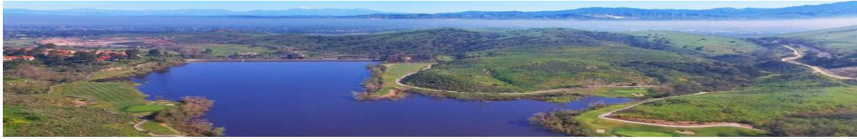
Figure 8.11: The Sand Canyon effluent storage reservoir at the Irvine Ranch Water District in California, USA
