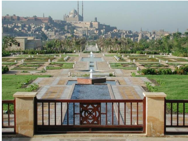
Figure 81 Using multiple levels to show the aesthetics of the Al-Azhar Park Source: Saleh, 2018
