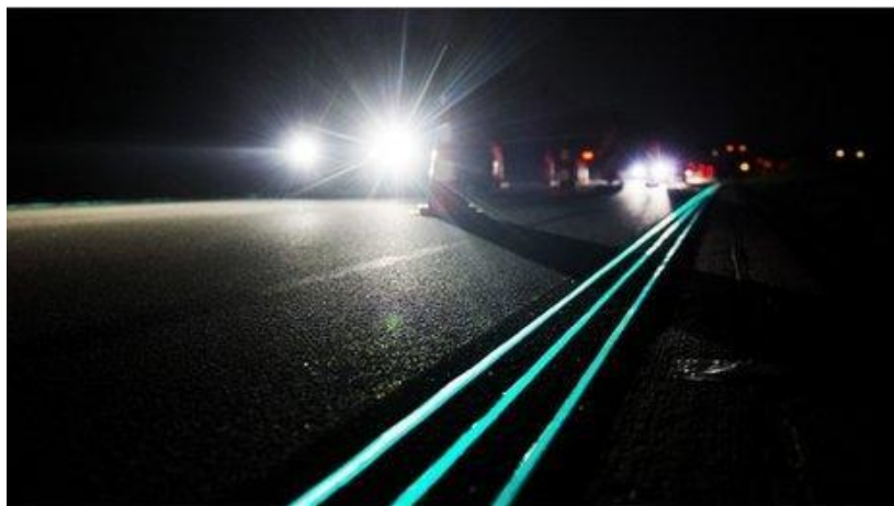
Figure 1.2. Glow in the dark roads near Oss in the Netherlands. The road marking absorb light during the day and emit the green glow at night providing visible trajectory lines to road users. Adapted from Scott [29]. Copyright 2022, National Public radio NPR.
