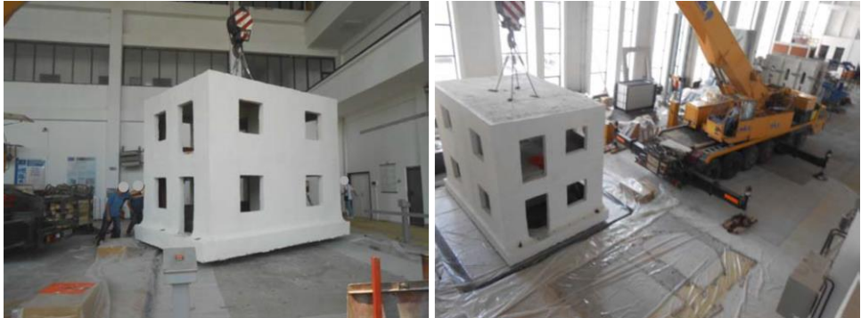
Figure 6.8: Transportation of the BM-SR model and positioning on the shaking table [73]
