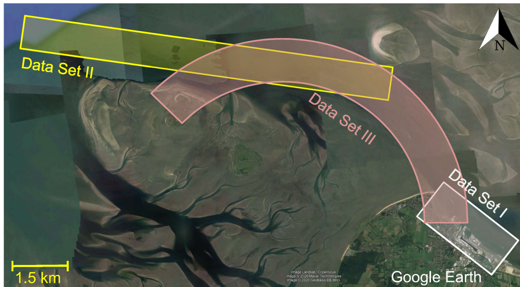
Figure 6.8: Google Earth image showing the test site in North Sea near Cuxhaven, Germany. The data sets marked in the figure are described in Table B.2 (cf. page 151).
