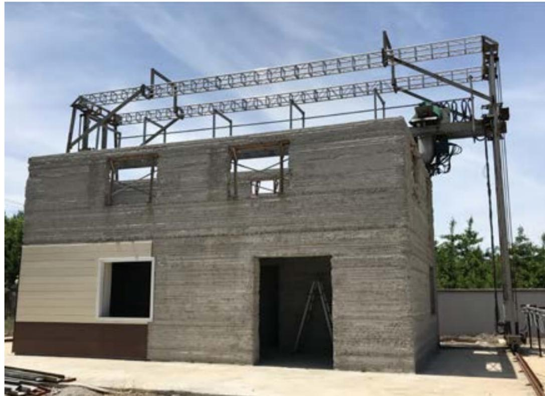
sector are primarily concentrated on concrete as a material. Thus, at the international level, there is a rapid increase in demonstration projects for 3D concrete printing of mostly small buildings. And in Germany as well, first pilot projects are being implemented.
