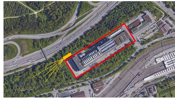
Figure 4: The "Geospeicher Forsthaus" is being built on the site of the Forsthaus energy center.
