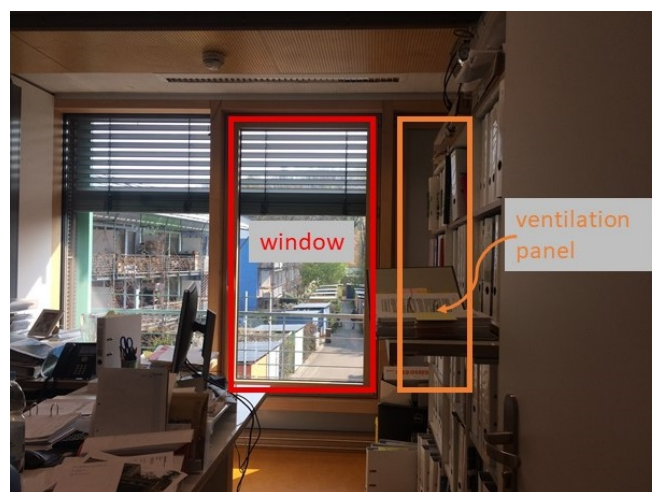
Figure 7. View into the investigated office room with highlighted window and ventilation panel [Fraunhofer ISE].
