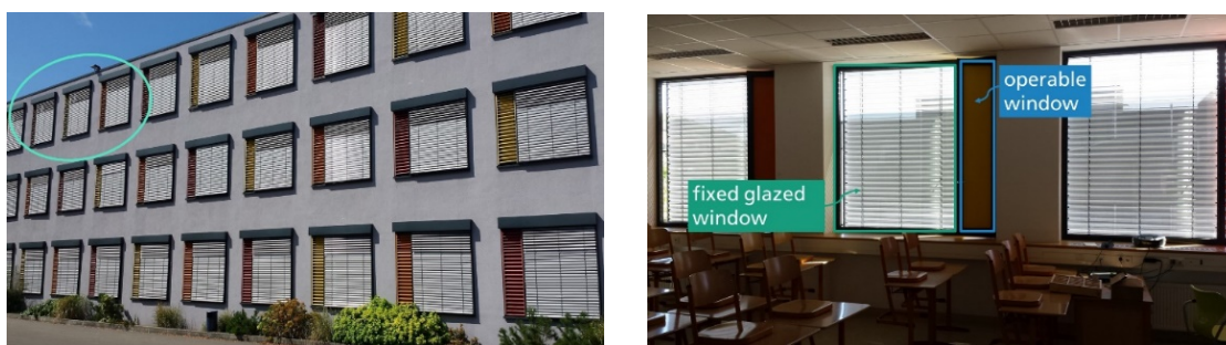
Figure 4. Left: View of the east façade of the school building. The examined room is marked in orange. Right: Interior view of the window front. The right wings of the windows can be opened, and permanent sun and rain protection is installed in front of them [Fraunhofer ISE].
