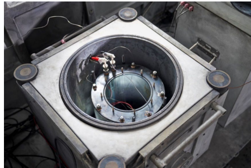
Large canister in EV+ ARC
