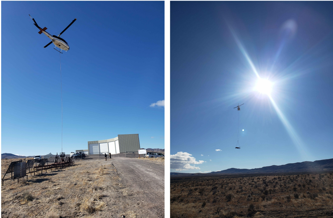
Figure A.7.: Pictures of the helicopter deploying the heavy components of the SAE station. Due to environmental protection, the field can not be accessed with trucks. A helicopter is used to bring the heavy components into the field. This includes the scintillator panels, the solar panels, the battery box and the antennas. Left: The components of the SAE waiting at the Middle Drum fluorescence detector for their deployment. Right: One of the scintillators being carried by the helicopter into the field [67].
