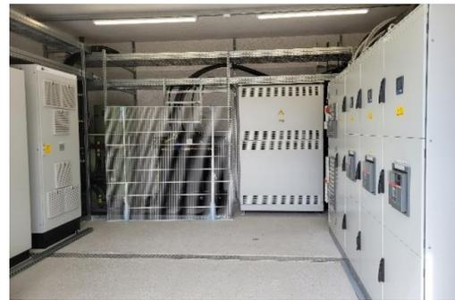
Figure 16 Upgraded power supply (transformers, rectifiers, power switches) for MEKKA and MaPLE in new building.
