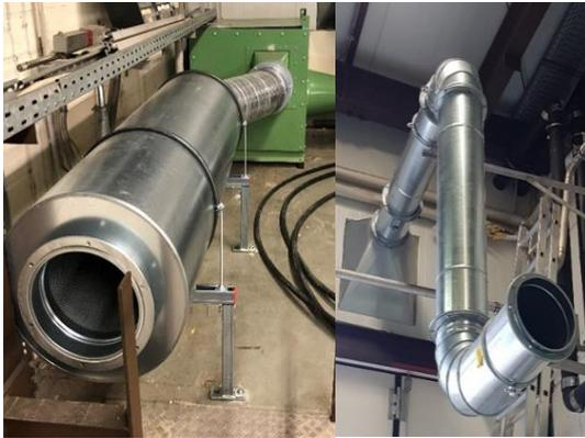
Figure 18 Air-blower fitted with new noise silencer and building lead-trough.
