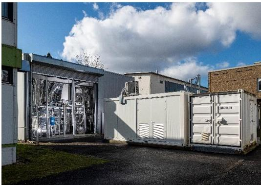
Figure 13: Demonstration plant built at KALLA: view of the entire plant: from left to right, the pyrolysis reactor with the container plants from INERATEC and Climeworks.
