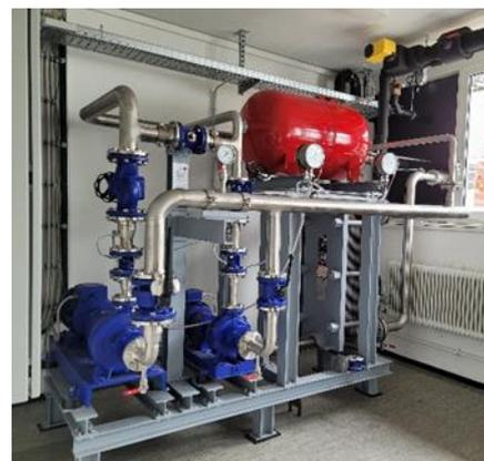
Figure 17 Pumps for water cooling circuits for MEKKA and MaPLE magnets at new location.
