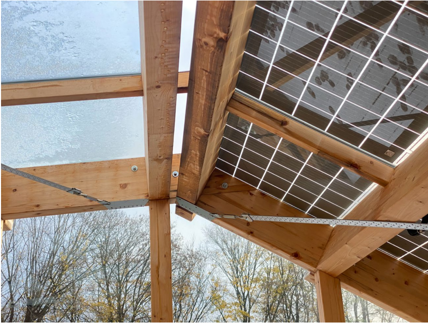
Abb. 121: Semitransparente Photovoltaik
