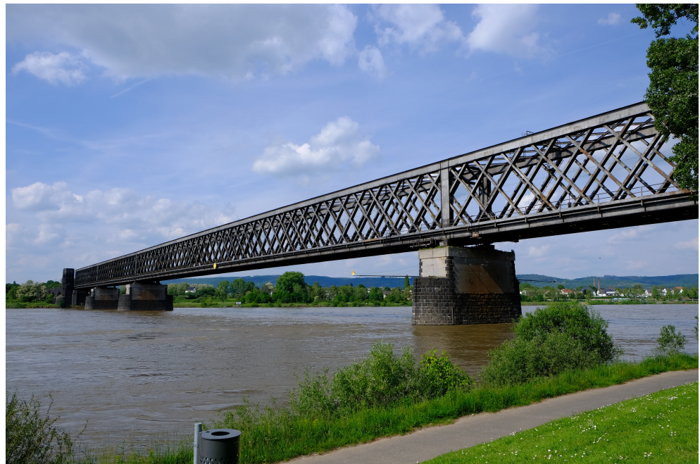
Figure 5. Railway framework bridge under investigation.
