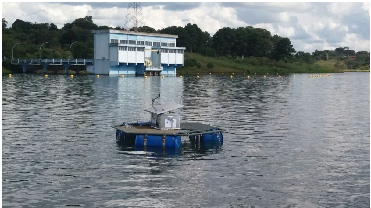
Figure 22 – Floating platform system located in Passauna reservoir next to the water intake
