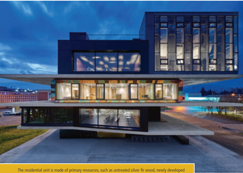
The residential unit is made of primary resources, such as untreated silver fir wood, newly developed construction materials, and recycled resources.
