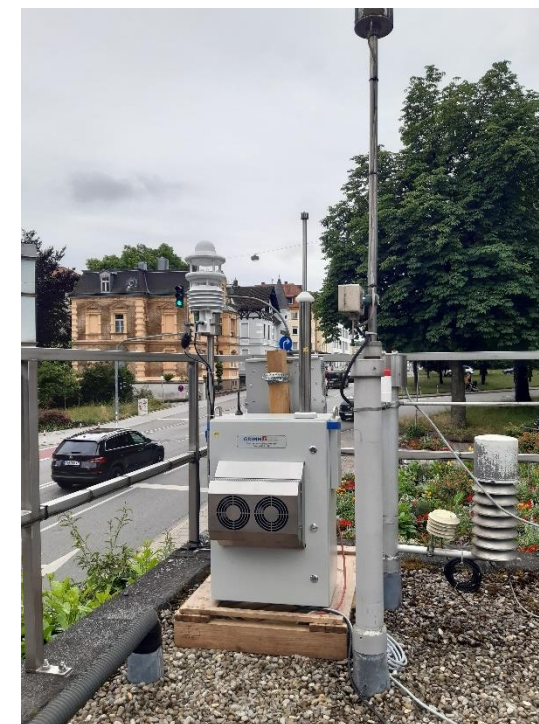
On the roof of the network station (LfU) in city center of Regensburg
