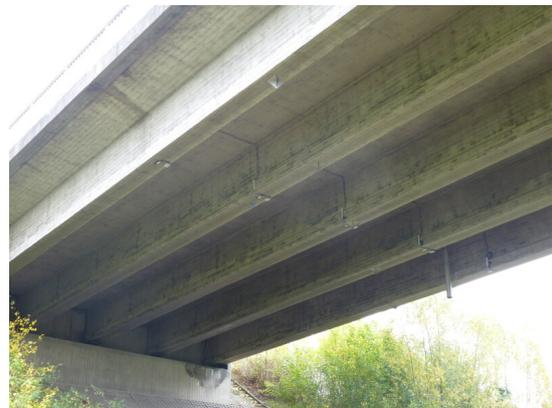
(f) Installed reflectors in Seßlach.
