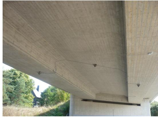
(b) Installed reflectors in Schneckenlohe.
