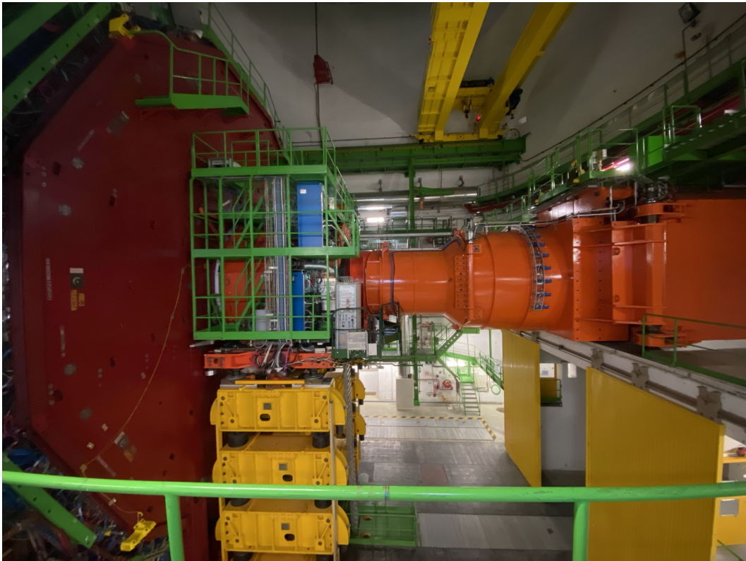
(a) Full closed CMS forward shield installed at present (in orange).
