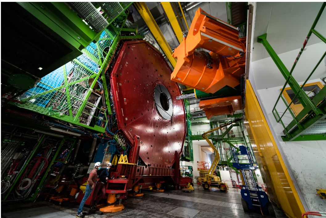
(b) CMS forward shield installed at present (in orange) during the full opening procedure [113].
