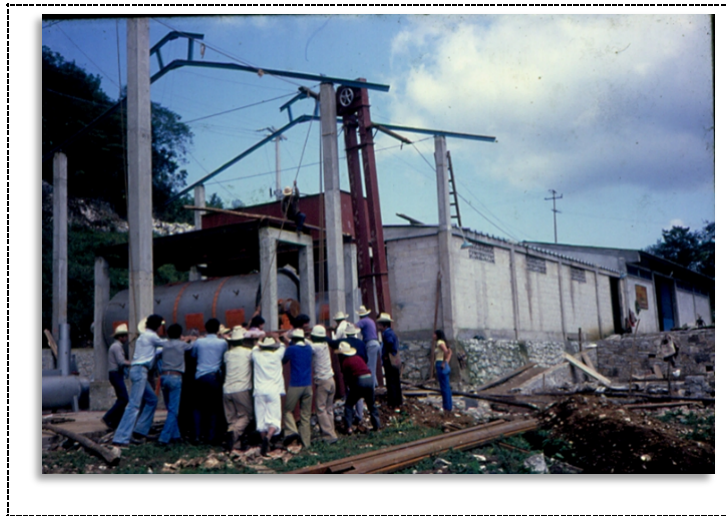
Figure 13. Community members taking part in 'Tequio' by building a civic center.
