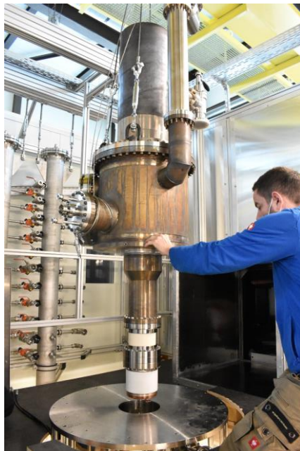
Fig. 1.3.2: Installation of a short pulse 1.5 MW 140 GHz gyrotron.
