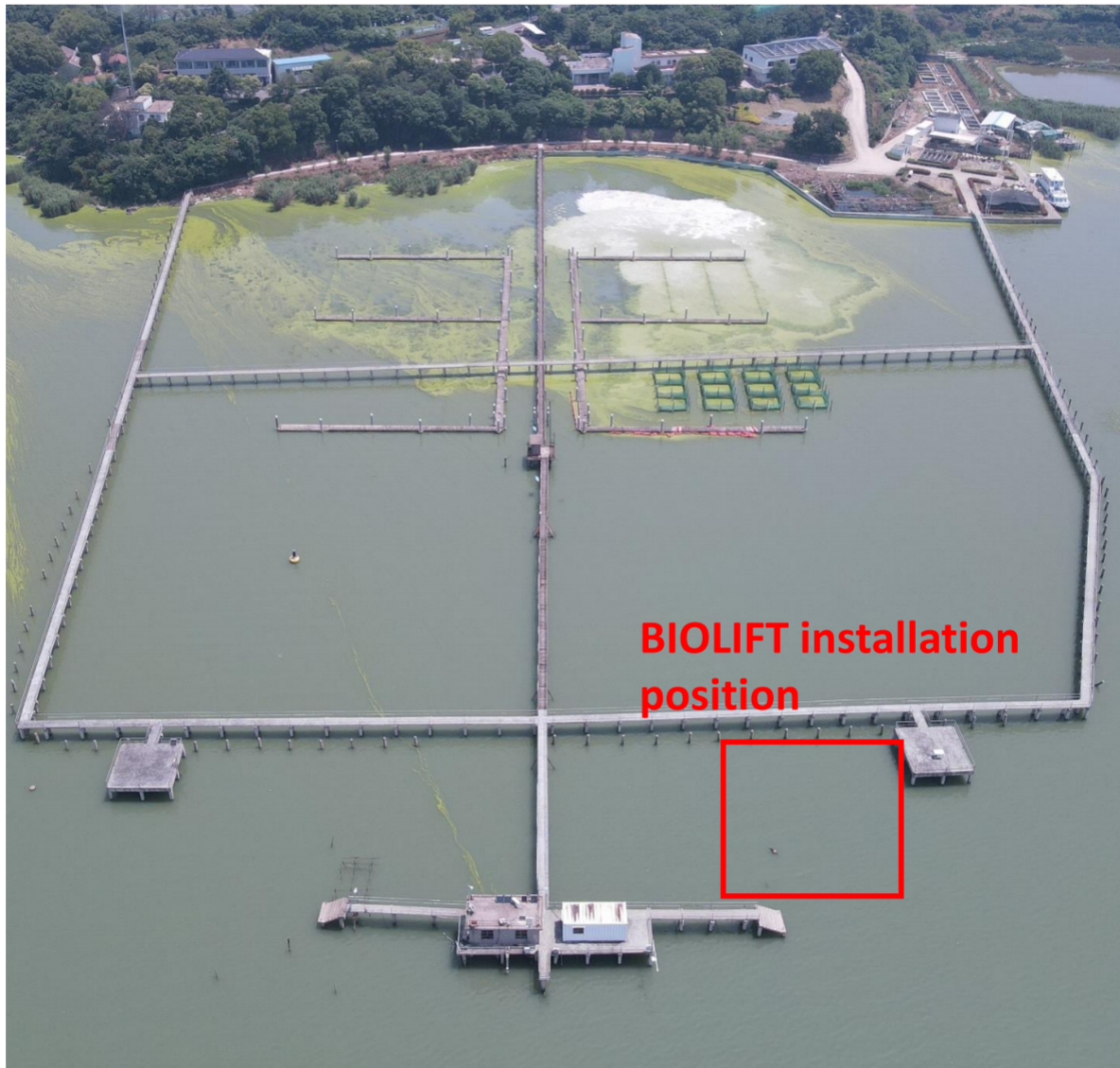
Figure 6.2: Panoramic photograph of the TLLER and the BIOLIFT installation position
