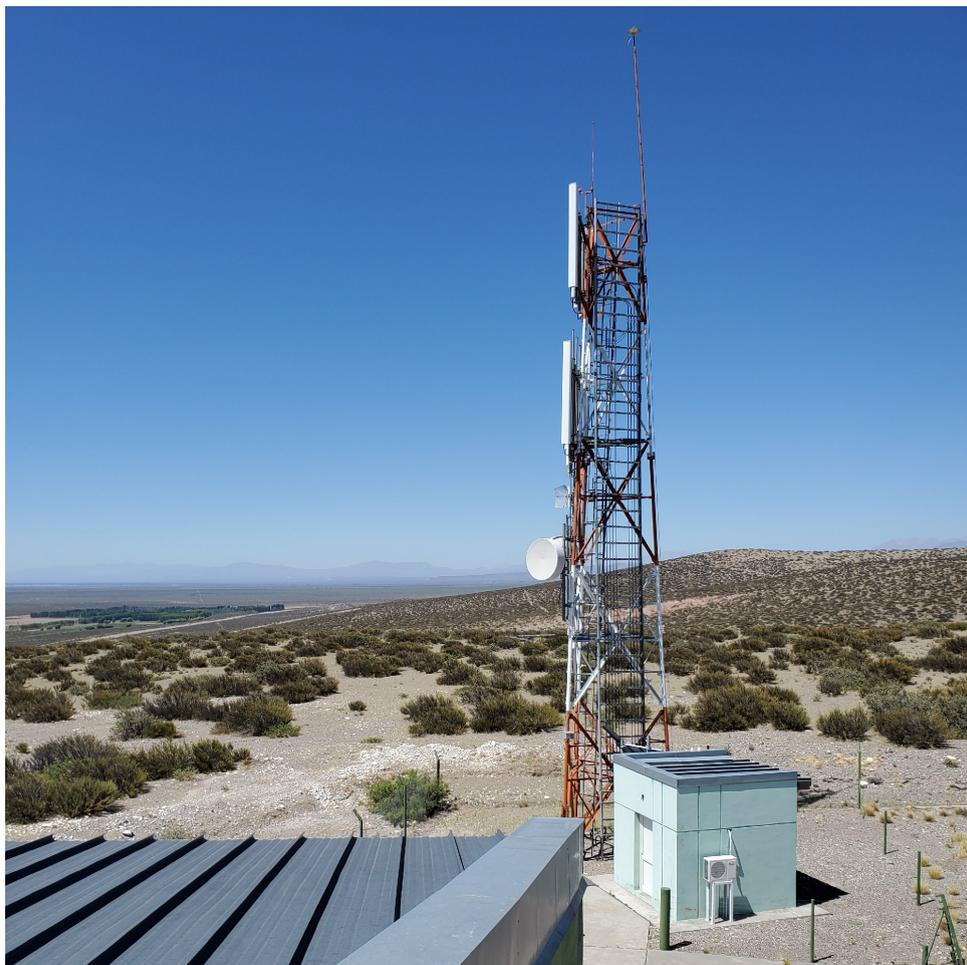
Figure 3.3: Photo of the Coihueco communications tower as viewed from the roof of the local FD building. Picture taken on 2022-08-30. Beacon dipole antenna visible below the white dish. For the mount location also refer to Fig. 3.4.
