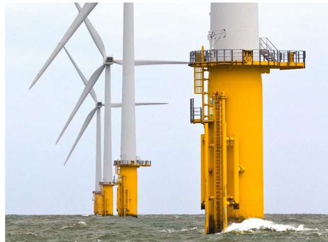
Figure 1 Offshore wind energy plant with secondary steel structures. Source: Mark Leybourne, CC BY 2.0, edited [1]
